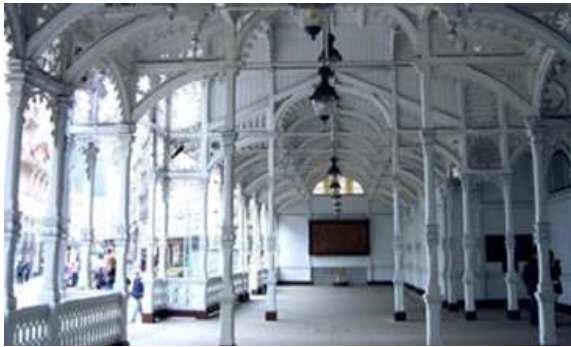
Fig. 2. Drinking water springs pavilion, Karlsbad/Karlovy Vary
