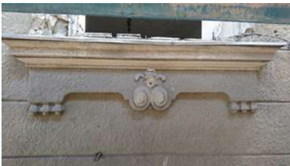
Fig. 10. D05, Solbanc window, floor II
