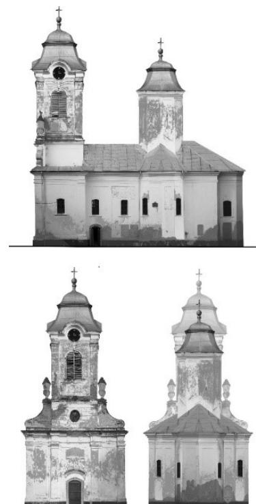
**Fig. 3.** 3D laser scanning of Bezdin church – façades
