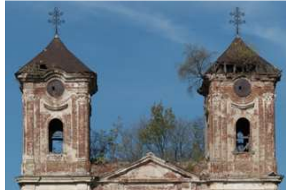
Fig. 10. Vegetation taking over where the roof used to be
