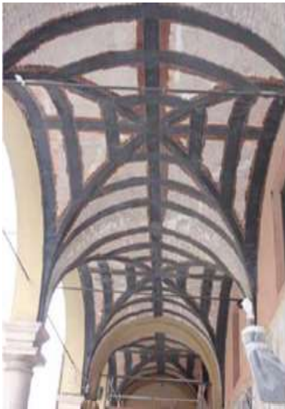
Fig. 19. Consolidation FRP of vaults [4]
