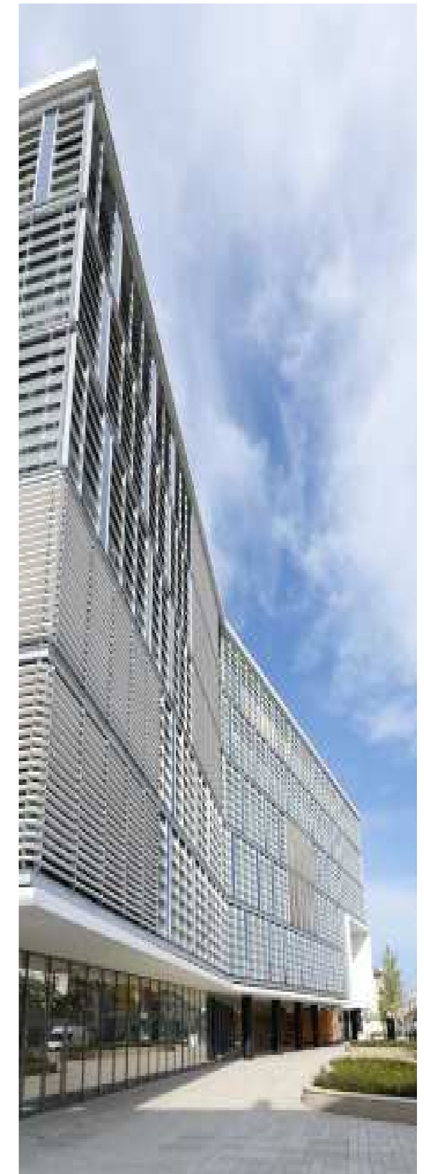
Fig. 10. Materiality - stone and glass THE OFFICE
