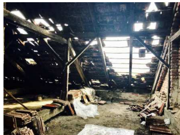
Fig. 4. Lajos Palace, the attic, existing situation
