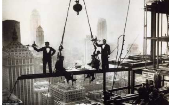
Fig. 8. Historical steel structures. Source: https://www.dailymail.co.uk/news/article-2920453/Laughing-face-death-Incredible-pictures-construction-workers-fooling-built-America-s-iconic-buildings.html
