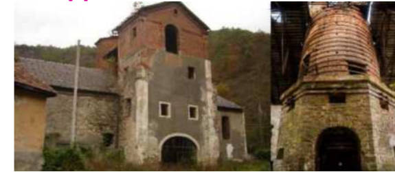
Fig. 2. The furnace in present - exterior and interior view (2016)
