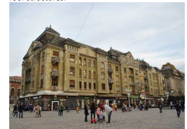
Fig. 2. Roof structure with a significant role in defining the urban context
