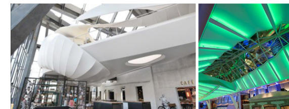
Fig. 12. Suspended PVC installations [23]
